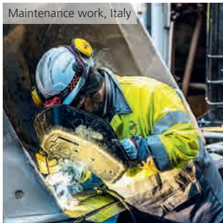
Maintenance work, Italy
