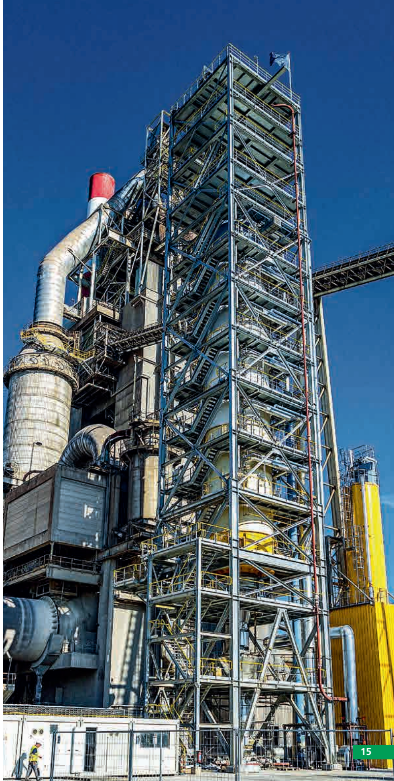
Right: Carbon capture with LEILAC technology at the Lixhe cement plant, Belgium
